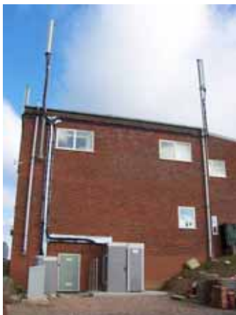
Antennae pole mounted to side of building
