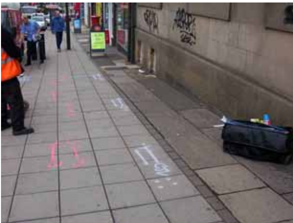
Street works installation - pre start
