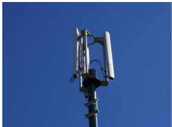
Greenfield column head frame - close view
