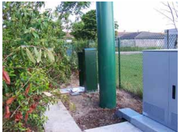
Greenfield cabinets and column reinstatement
