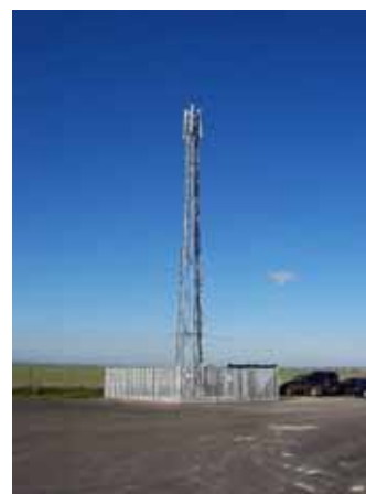
Greenfield macro site completed
