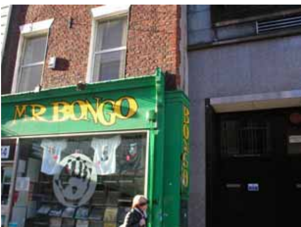
Micro cell decommission - before
