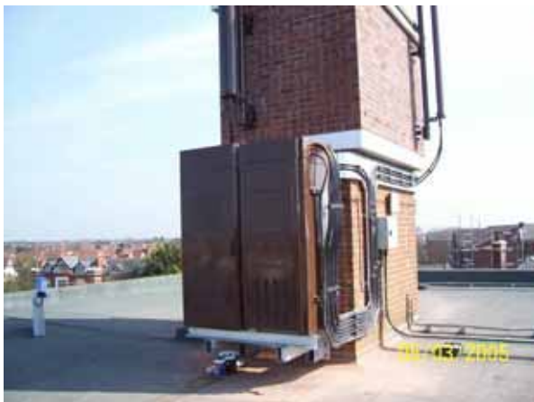
RF equipment installed on steelwork mounted onto existing structure
