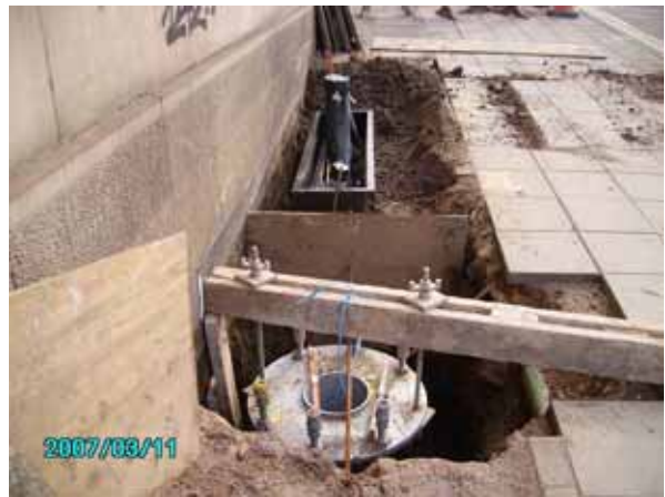
Street works installation - root section install
