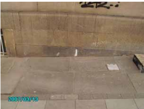
Street works installation - interim reinstatement
