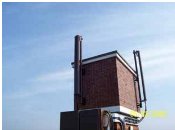
Panel antennas installed onto existing structure
