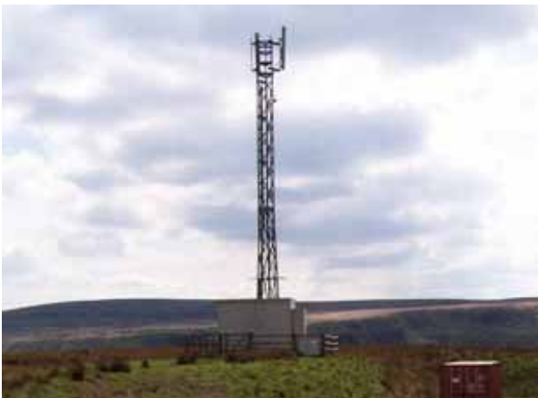
Macro greenfield site decommission - before
