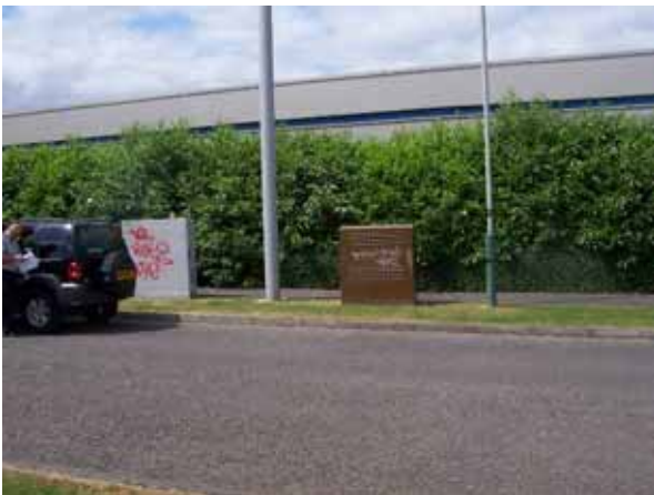
Upgrade of UMTS equipment - before
