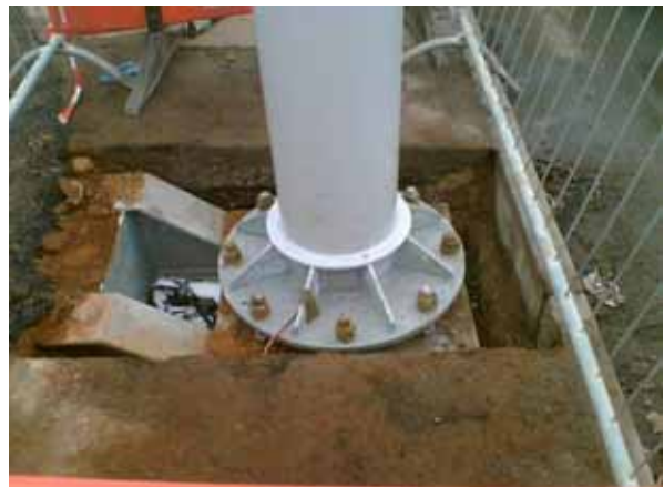
Column installed onto additional root section
