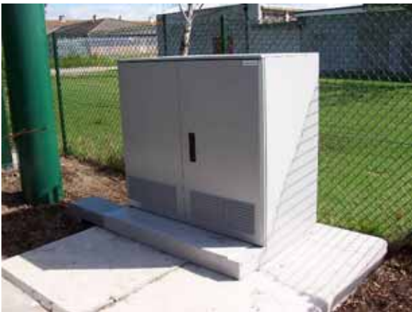
Greenfield cabinet installed on concrete base
