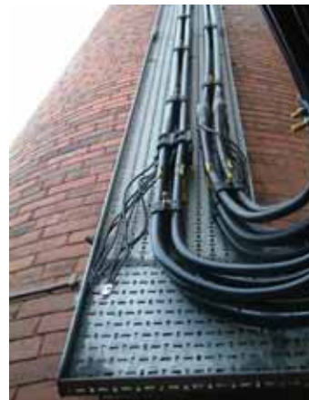
Feeder cables fed onto cable management system
