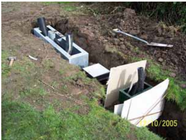
Cabinet root sections prior to concrete pour
