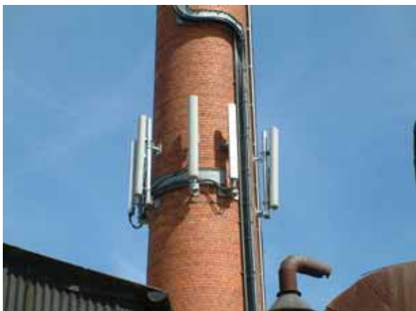
Antennae mounted onto existing chimney stack
