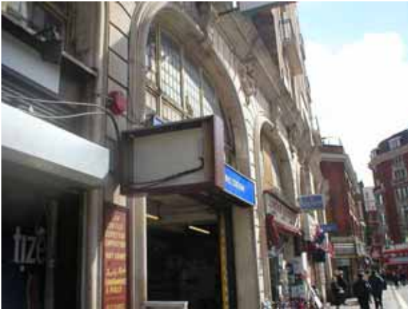
Antenna installed in sign to reduce visual impact
