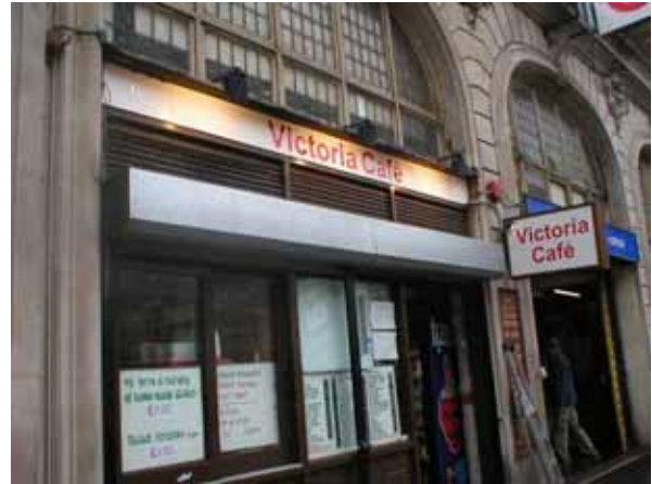
View of site once all works have been completed
