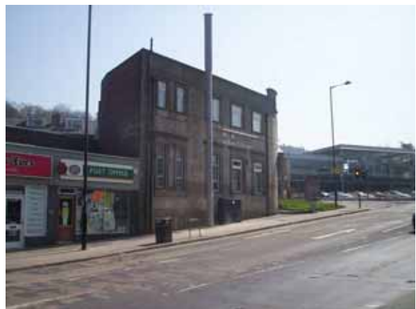
Street works installation - completed site
