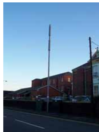
Upgrade of column structure - after
