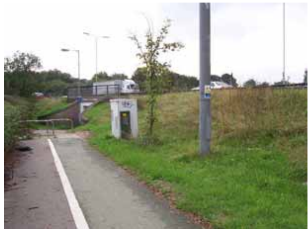
Monopole location prior to decommission
