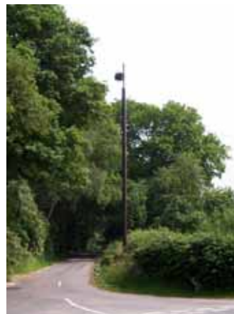
Microwave dish mount structure
