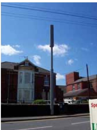
Upgrade of column structure - before
