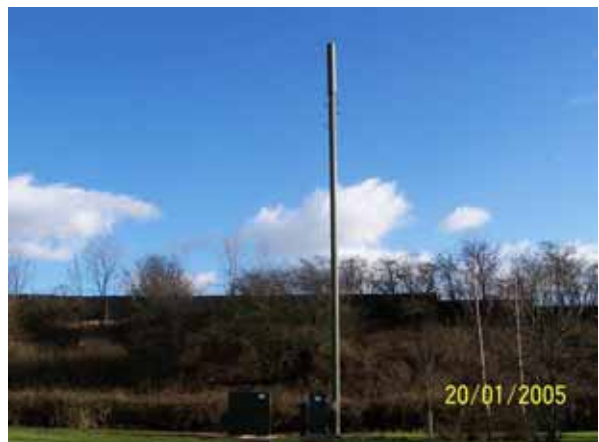
Completed site view
