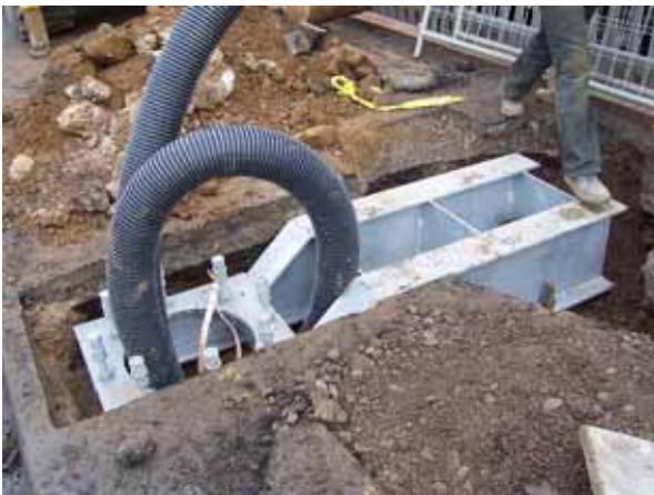
Additional root section used to avoid services
