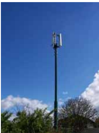
Greenfield column head frame - long view
